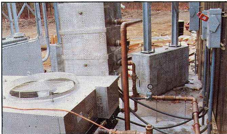
At one end of the heat exchanger system, coolant plumbing, pressure monitoring and pump powering arrangements are visible.
